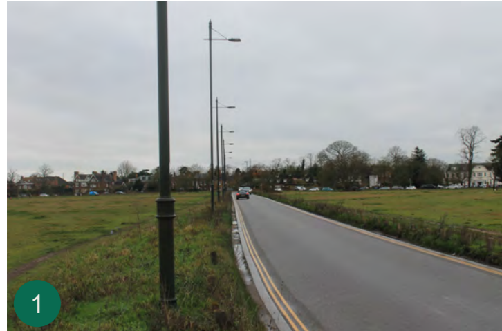
1 Cannizaro Road running through Rushmere. The existing meadow buffers on either side of the road are very narrow
