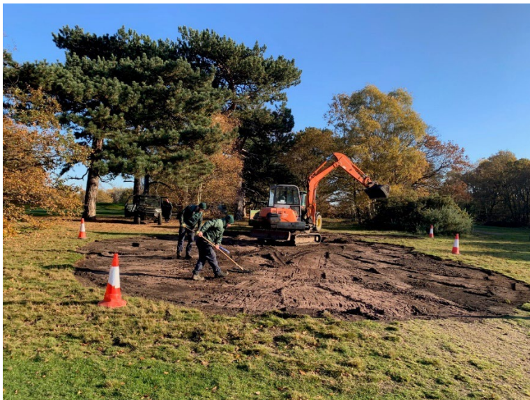
Birches Fairway bare ground creation site
