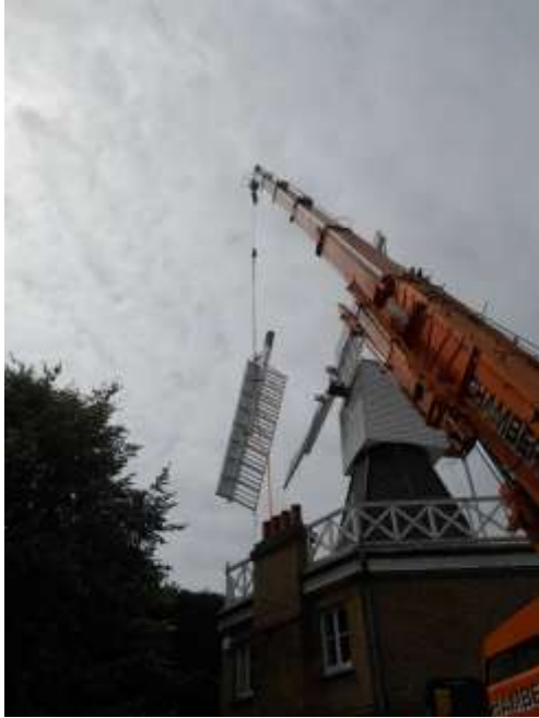
The sails being removed from the Windmill
